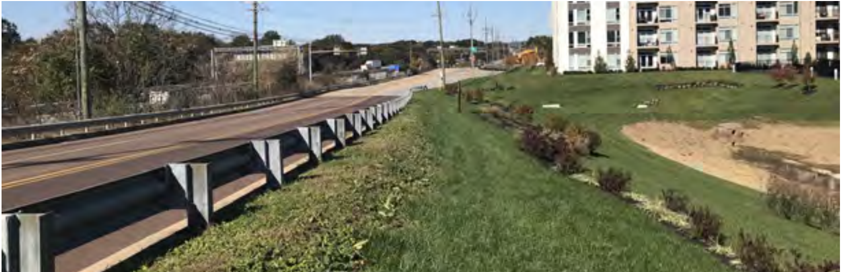
Guthrie Road - existing conditions
