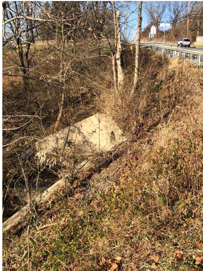
North Gulph Road over Trout Creek. Alternative 2A would extend this culvert to accommodate the trail; Alternative 2B would construct a separate bridge just west of the culvert.
