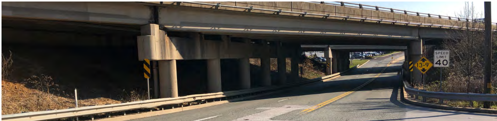
The US 422 bridges over North Gulph Road
