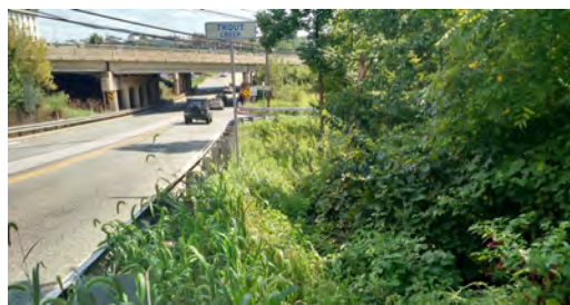
North Gulph Road crossing Trout Creek
