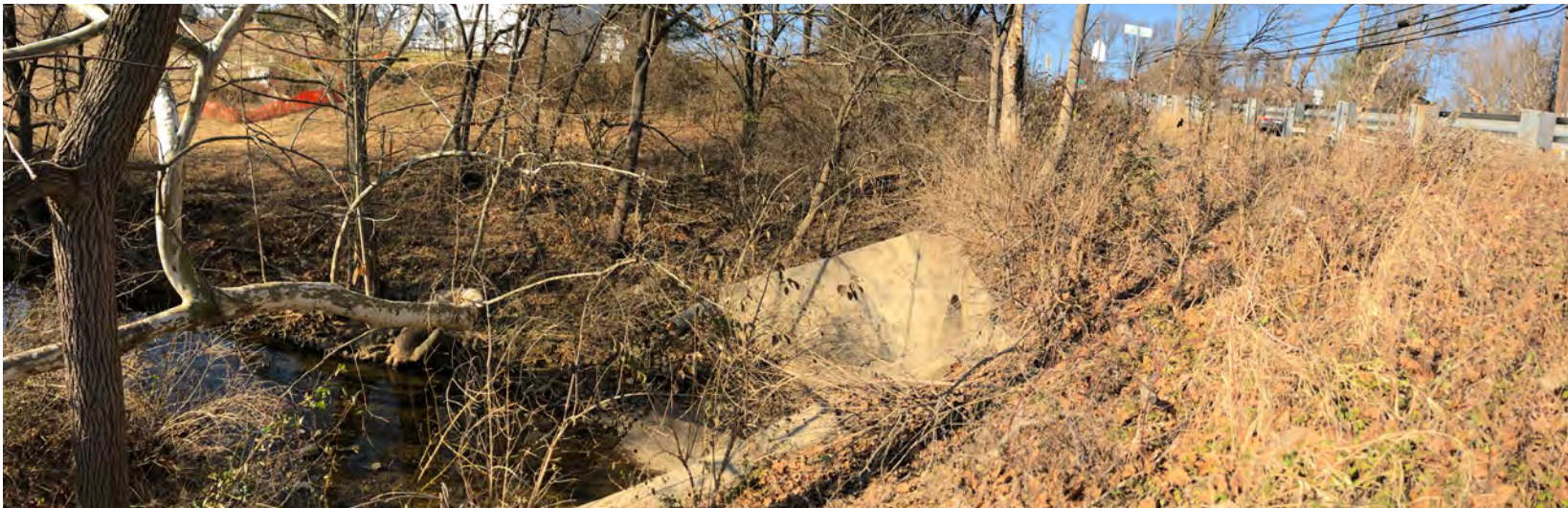
Trout Creek culvert (looking north)
