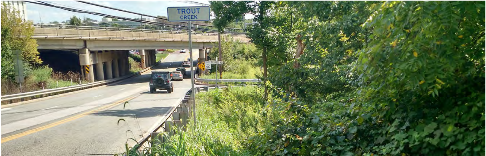
North Gulph Road at Trout Creek (looking south)
