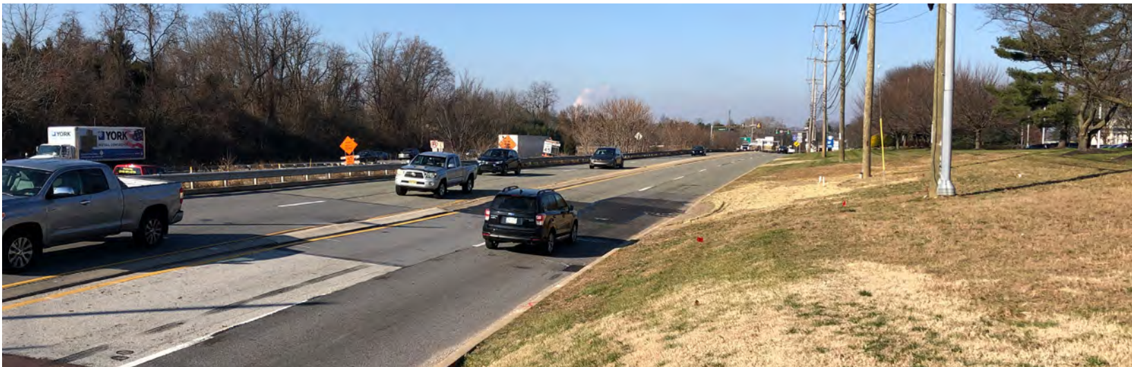
North Gulph Road at the Pennsylvania Turnpike (looking north)
